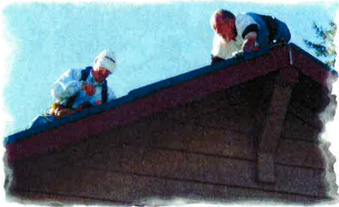
SOWERS finishing up the roof project
